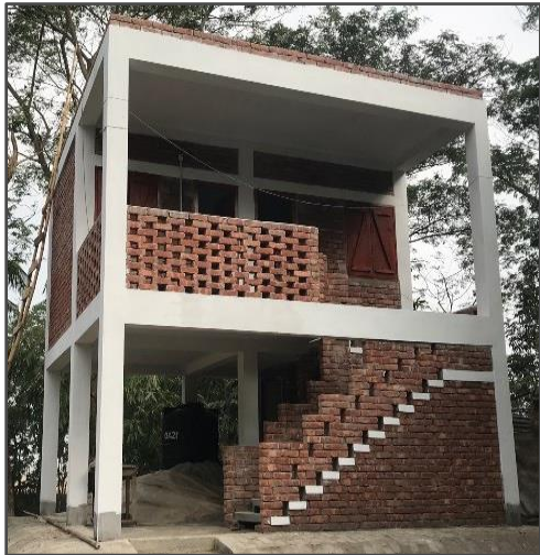
Improving resilience to intensifying cyclones and heat stress through modified and improved shelters/structures
